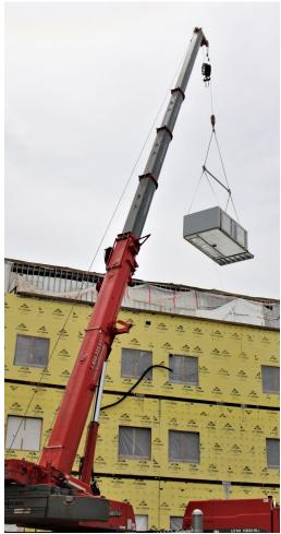
The "penthouse," or the top floor of the new wing, houses the heating and cooling systems for the new construction, as well as parts of the existing building. This includes air handlers, chillers, boilers, and energy recovery units.
