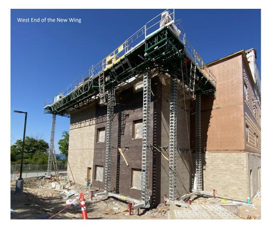
The exterior façade of the Offield Family Pavilion is in various stages of completion. Application of the clay-colored sealant over the yellow insulation board is nearly finished.
